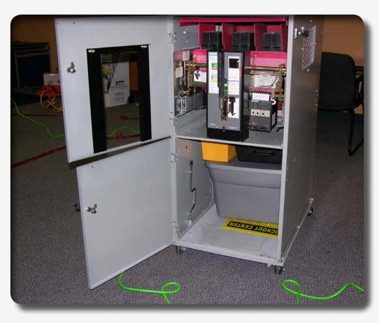
Students practice voltage testing, proper barricading techniques, and installing grounds and grounding clusters, on the NTT designed hands-on training equipment. This specially designed equipment allows students to remove and re-install (rack in and out) draw out type circuit breakers. It incorporates a visual indicator to ensure proper position of the breaker in the cubicle. Students wear proper PPE for these tasks and utilize live line tools.
